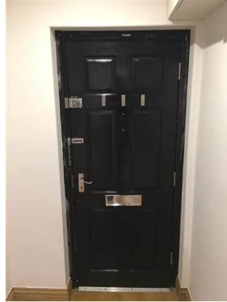
Interior door. I to match exterior. Paint marks and small chips in places. Chrome effect chain lock Wear and tear
