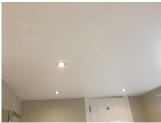
Ceilings painted white x8 spotlights, LED bulbs all working
