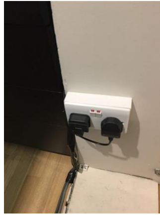
Double socket TV cables connected
