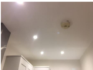
Ceiling freshly painted white
