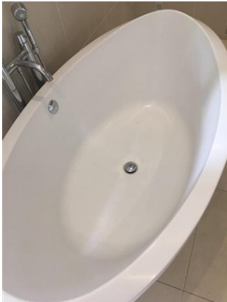
PVC bathtub with chrome pop up waste Some scratches in places Wear and tear Floor mount mixer tap, flexible hose with shower head - not working
